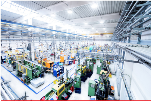
Power & Control Systems
